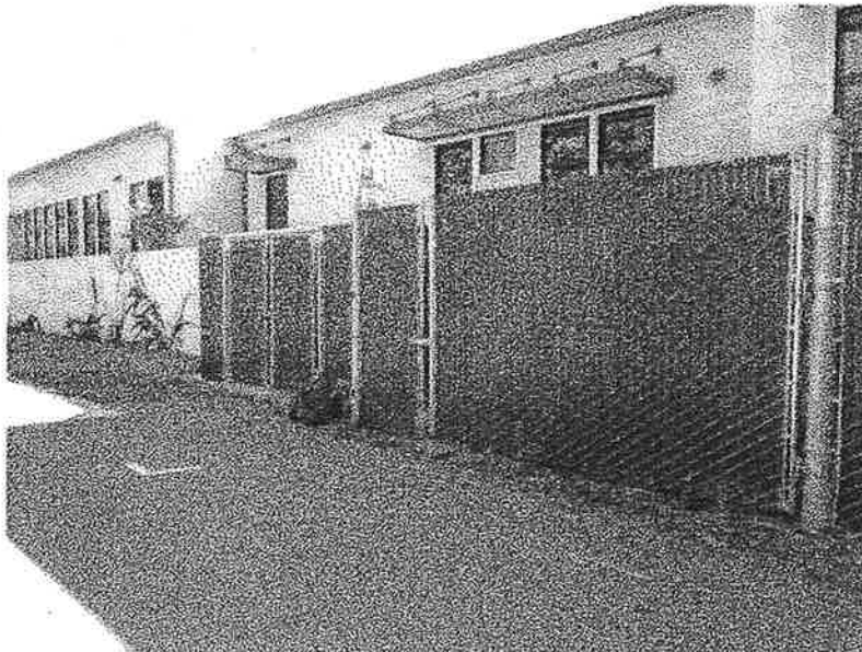
Transformer/equipment enclosure (Middle School in background) SW corner
