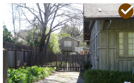
Locate an Accessory Dwelling Unit (ADU) to be subordinate to the primary structure.
