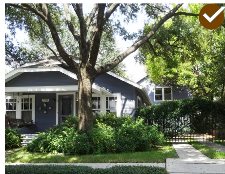
Locate a secondary structure to be subordinate to the primary structure.
