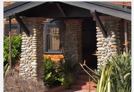
Masonry, such as stone or brick
