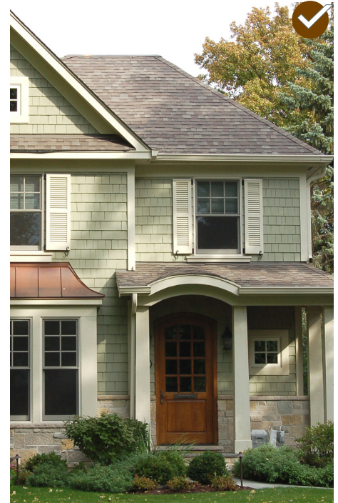
Size a door to be easily readable and recognizable, but not to be overly large.
