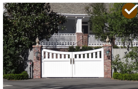
Design the vehicular gate to be low in scale to maintain the visual connection between the public and private realms.
