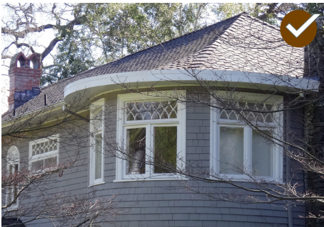
Size and proportion a window to be in the range of heights and widths of windows seen traditionally in the block.
