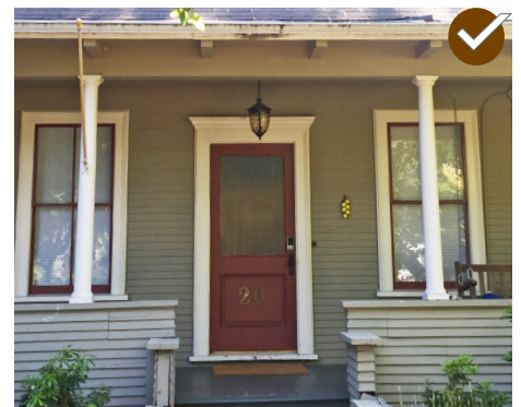
Use an architectural element, such as a stoop or porch, to highlight an entrance.
