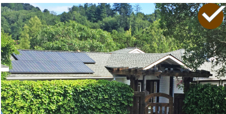
Locate attached or detached solar technologies, such as solar panels and solar cells, where sun will be harvested, as well as where technologies are least visible from the public realm.
