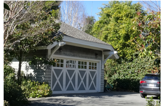
*Garage is seen from the alley in this photo.
