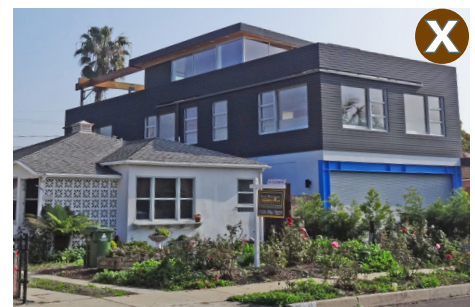
Where a building is located near a shared rear or side lot line, variation in massing may be particularly important to avoid looming impacts.
