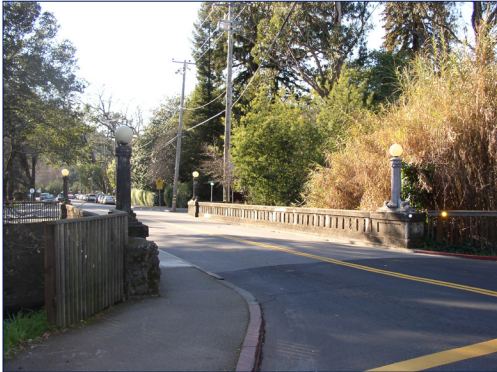
Lagunitas Road/Lagunitas Bridge entryway to Ross
