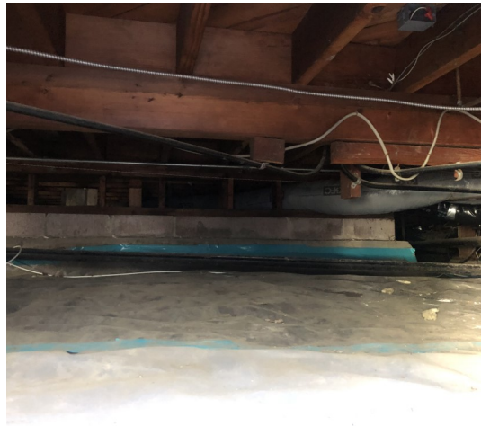
Under floor of Police Station
