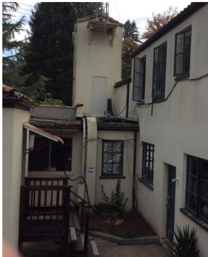
Image 6: Infill between central and north wing
