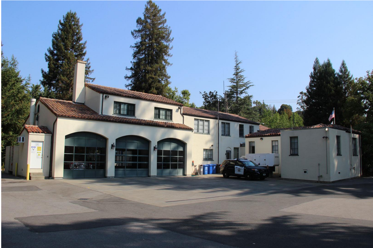
Figure 17. South façade of firehouse.
