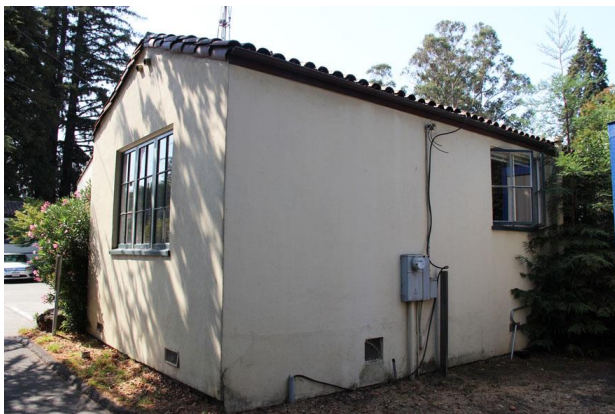
Figure 23. Part of the north façade of north wing.
