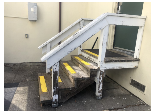
Police Station exit stairs
