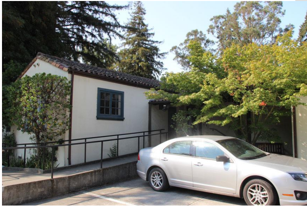
Figure 12. North and east façades of south wing.
