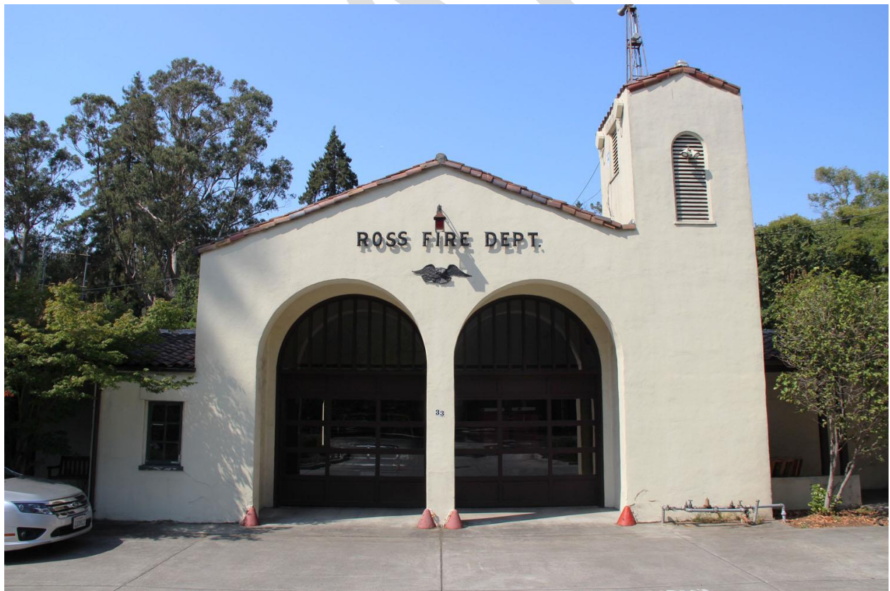
Figure 16. East façade of firehouse.
