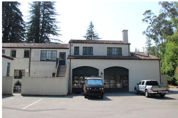
Figure 19. North façade of firehouse addition.
