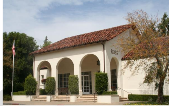
Figure 3. Ross Post Office; view toward northeast
