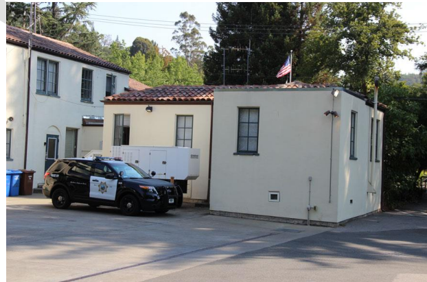
Figure 15. South and west façades of south wing.
