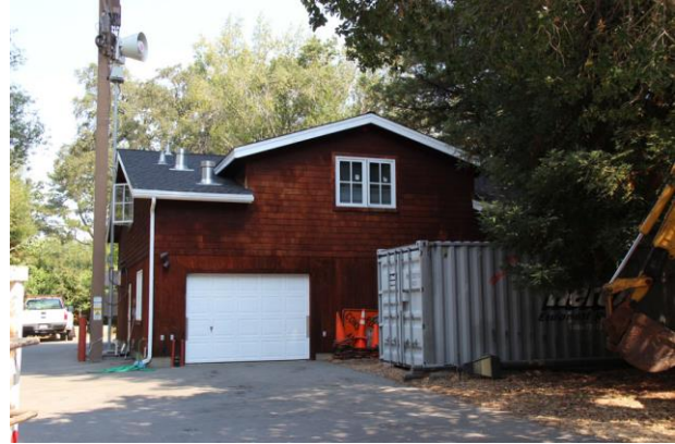
Figure 10. Ross Corporation Yard; view toward north.
