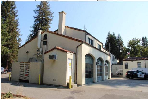
Figure 18. West façade of firehouse.
