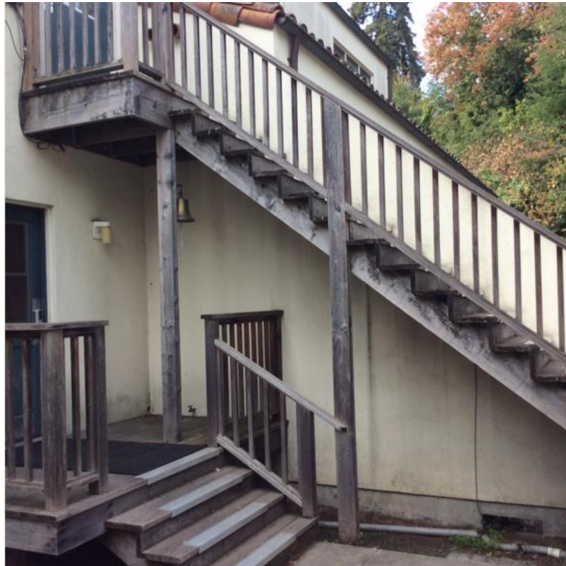
Image 8: Central firehouse dorm access stair (residential construction)
