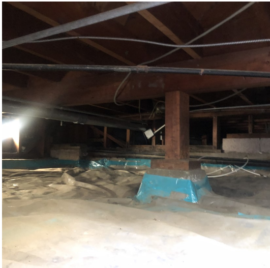
Under floor of Police Station
