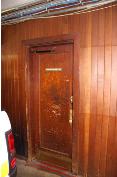
Figure 29. Redwood paneling in firehouse.
