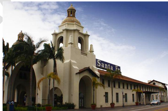
Figure 40. Santa Fe Depot, San Diego
