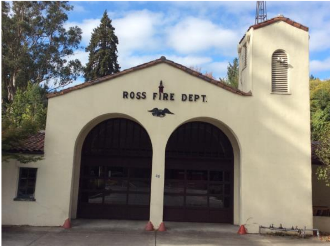
Image 1 Original Central Firehouse – Front elevation
