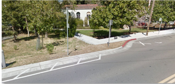
2 Westbound sidewalk gap on Lagunitas Rd.
