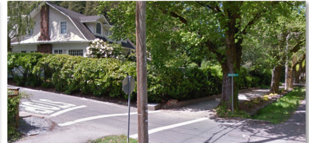
6 Unpaved walkway gaps on Lagunitas Rd.
