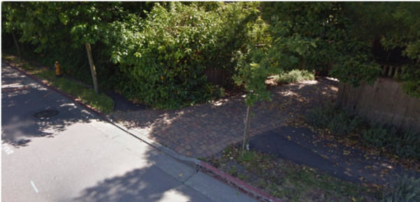
4 Southbound sidewalk gap on Poplar Ave.
