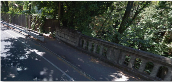
1 Southbound sidewalk gap on SFD Blvd.
