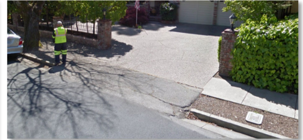
3 Southbound sidewalk gap on Redwood Dr.
