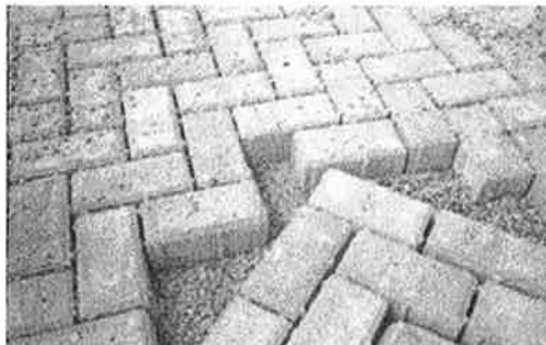
These heavy duty permeable pavers were used for a container port application in Latin America.
