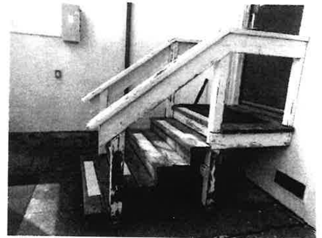
Police Station exit stairs
