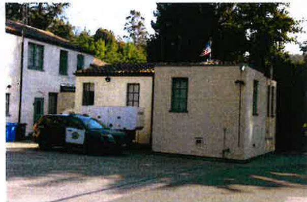
Figure 15. South and west façades of south wing.
