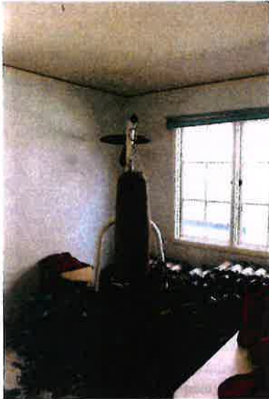
Figure 36. Bedroom in north wing.
