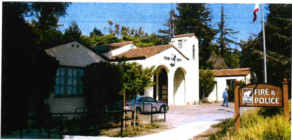
Figure 11. East façade of the Ross Public Safety Building; south wing at left, firehouse at center, and north wing at right.
