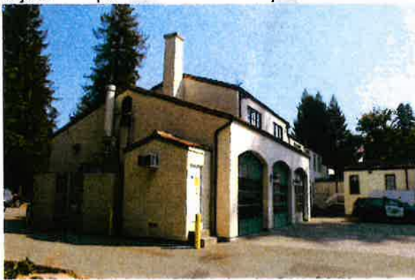
Figure 18. West façade of firehouse.
