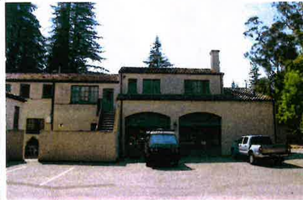
Figure 19. North façade of firehouse addition.
