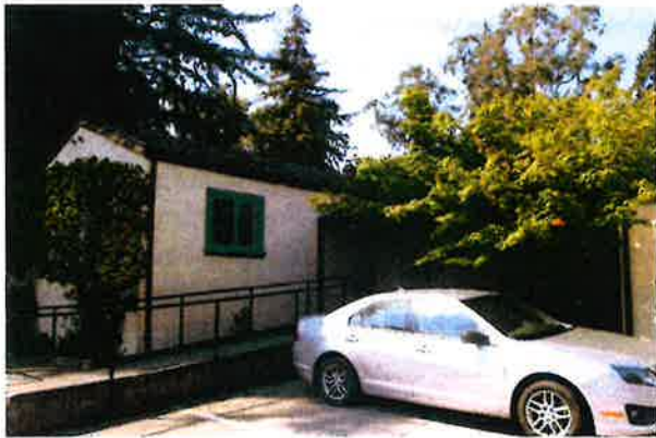
Figure 12. North and east façades of south wing.
