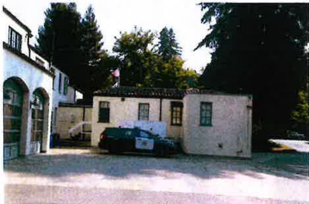
Figure 14. West façade of south wing.
