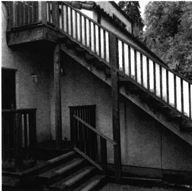
Image 8: Central firehouse dorm access stair (residential construction)
