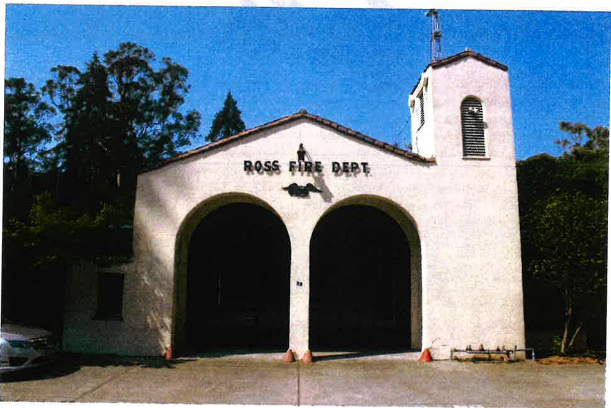
Figure 16. East façade of firehouse.
