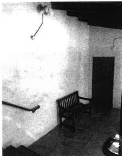
Faded plaster paint
