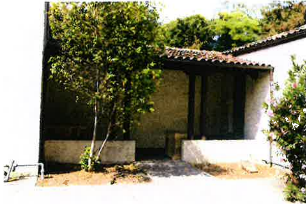
Figure 21. Hyphen and porch connecting north wing to firehouse.
