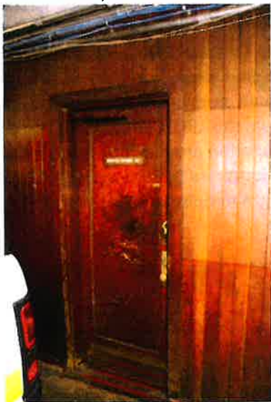
Figure 29. Redwood paneling in firehouse.
