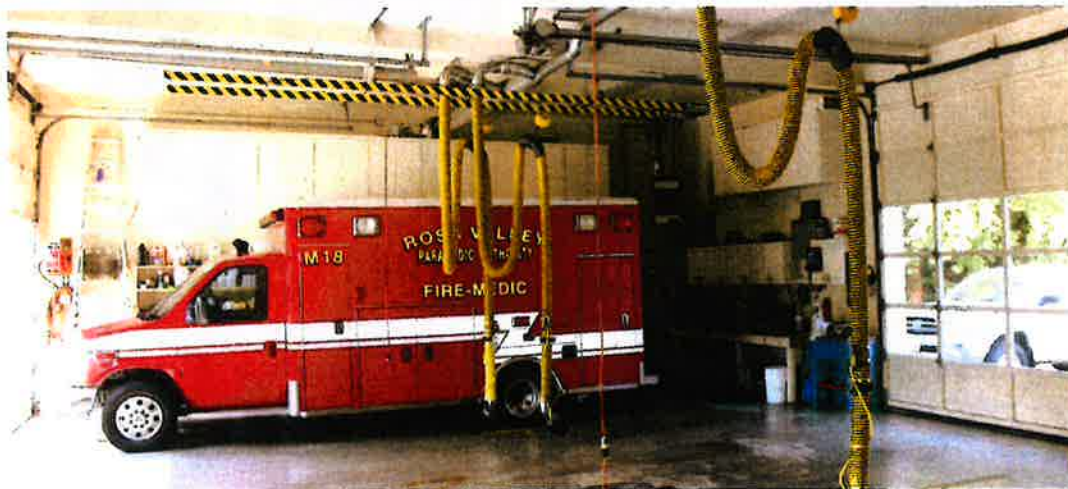
Figure 32. Vehicle bays in ca. 1995 addition.
