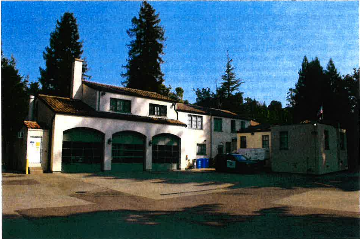
Figure 17. South façade of firehouse.
