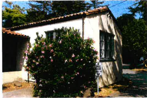
Figure 22. South and east façades of north wing.
